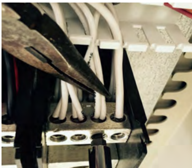
6) Secure line side L1, L2, L3 & Neutral wires to the top of the Distribution Blocks labeled L1, L2, L2 & N.
