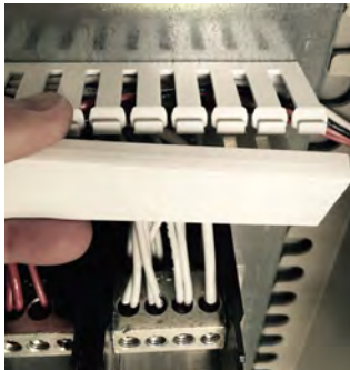
1) Remove wire raceway cover.
