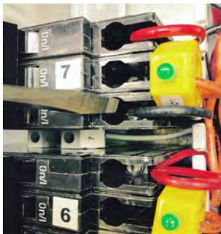
5) Secure the line side wires L1, L2, L3 to the top of the Breaker looping the L2 (Center Wire) through the LED Current Indicator.
