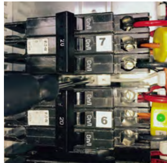
3) Secure the line side Neutral wire to the terminal block.
