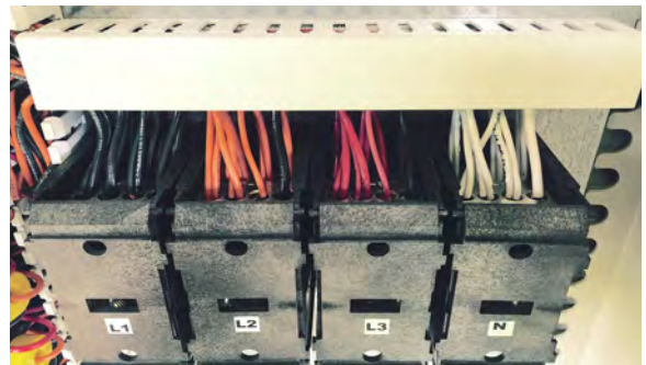
7) Replace the wire raceway cover.
